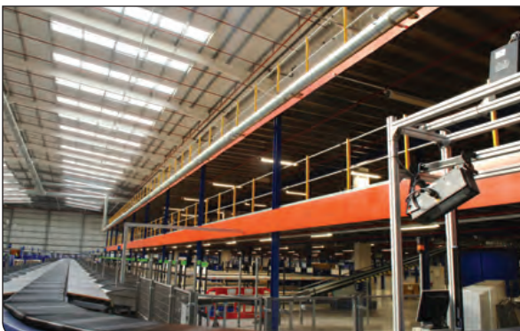
Mezzanines can be designed to accommodate a further floor at a later date future proofing the installation against planned growth.
